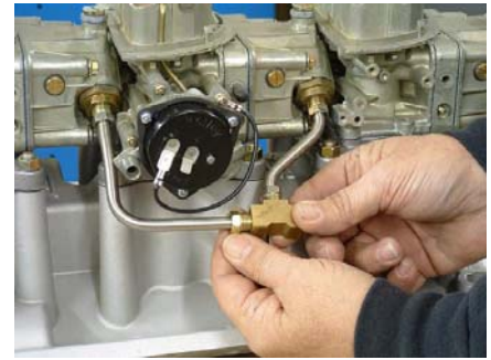
9: Continue installing fuel lines.
