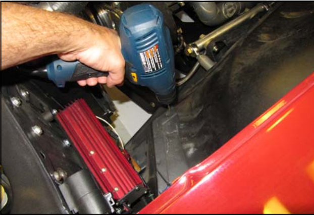
10. Drill 1/8" pilot holes into the inner fender.
