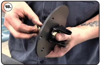
**18.** Insert a 1/2"-13 x 1 1/2" bolt through each hole of the flange/mount. The bolts need to be installed with the bolt head in the upper bracket. Refer to **Images 18 & 19**.
