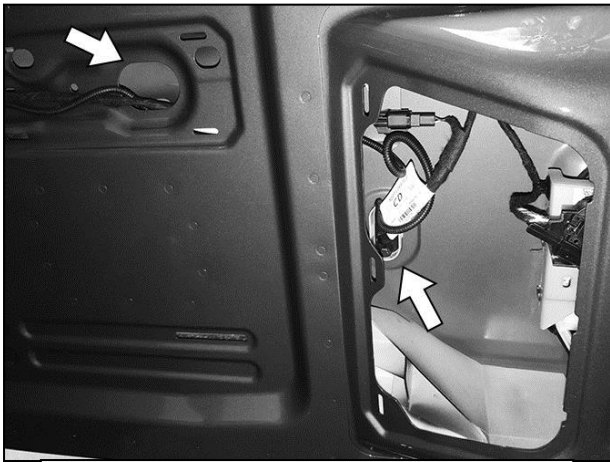
(Fig 19) Remove the plastic covers from the rear door. Feed Light Harness along the factory harness and out through the rubber plug in the door (arrows).
