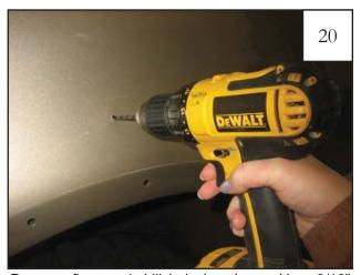
Remove flare and drill hole locations with a 3/16" drill bit, making sure to keep the drill level and perpendicular to fender surface.
