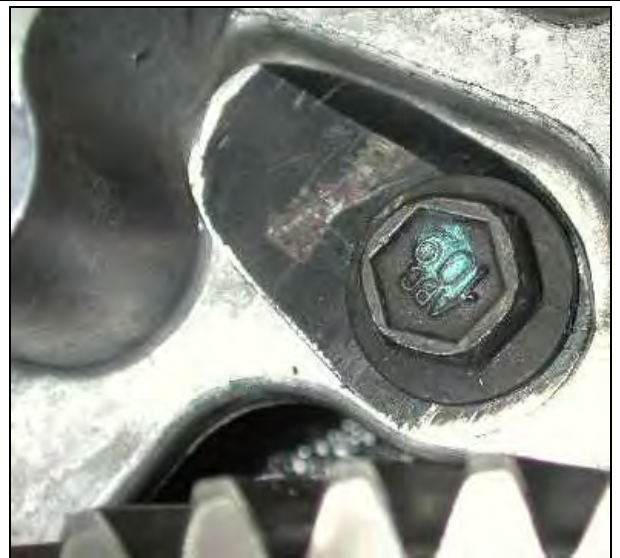
With retainer and bolt installed
