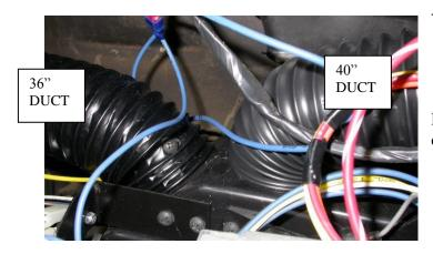
Route flex hose from right louver to top of distribution assembly.
