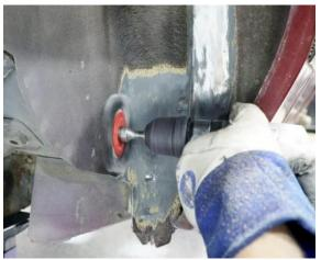
Figure 10 - Locate Spot Welds
