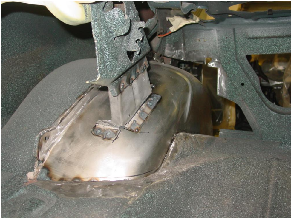
Figure 13 - Welded View (Trunk Area)
