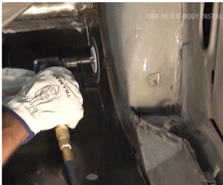
Figure 14 – Cut 1-1/4" Marked Lines
