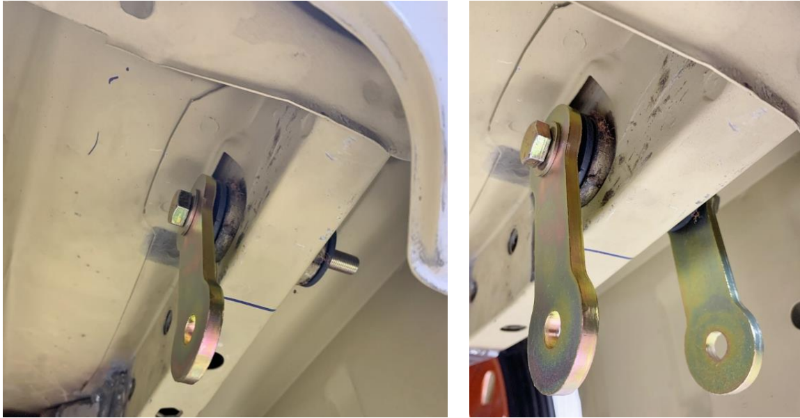
Figure 2 - Rear Leaf Spring Shackles Installed
