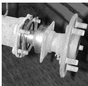
Installation of Spacer Plate.
