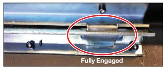
Close up of a hinge tab fully engaged.
