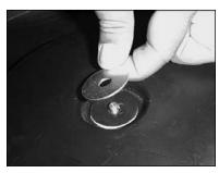
11) Place the provided large metal washer onto the stud.
