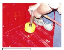
4. Mark the bed floor where the stack is resting. This is where the **Extension Pipe** will pass through the floor. Remove the stack from the bed of the truck. Find the center of the circle traced onto the bed floor, mark and center punch it. Drill the hole using a 5" hole saw. It may be required to cut part of a bed floor rail away. **See Figure 4.**
