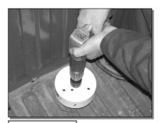
6. Cut a hole through the truck bed providing adequate clearance around the part of the "T" Pipe that passes through the truck bed. MBRP inc. recommends using a 5" diameter hole saw. It may be required to cut part of a bed rail away. See Figure 5.
