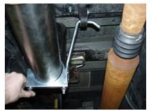
9. Install the **Hanger** by placing the **Plate Bolt** on top of the crossmember with the bolt extending down through the hole in the crossmember. Secure **Hanger** with 3/8" **Nut** and 3/8" **Lockwasher**. **See Figure 8**.
