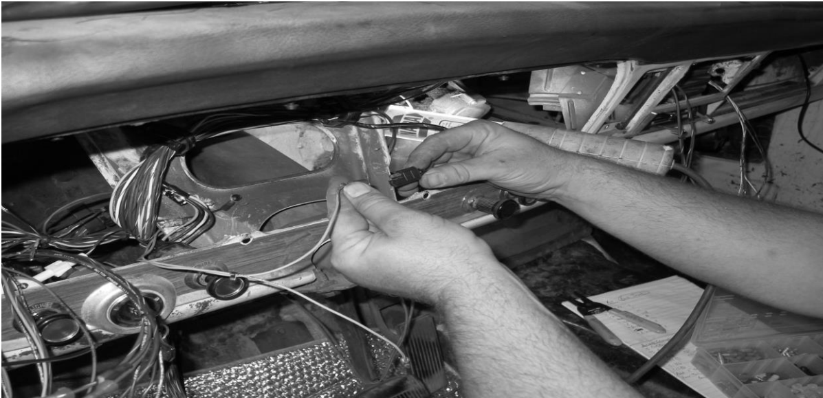
Figure 7-24 Cargo Light Connections
