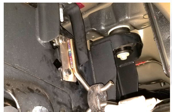
Detail 9: Frame hanger and grommet installed.
