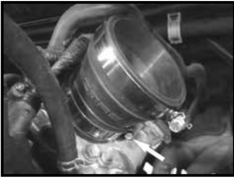
Step 8 Install new reducer coupler onto throttle housing and tighten one clamp.
