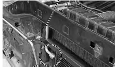
Install #8 Condenser/ Compressor Hardline onto #8 Condenser Fitting
