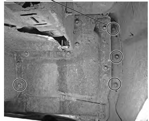
Passenger Side Fender View
