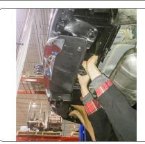
8. Secure provided fascia tab brackets to hitch main body plates, with 1/4" hardware, using 7/16 socket and 7/16" boxed end wrench. Align and secure (2) center fascia tabs by pushing nylon retainer clips into fascia tab brackets.
