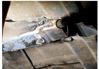
Figure 42 - Weld Back of Connector
