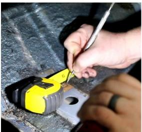
Figure 12 – Locate Cut Line
