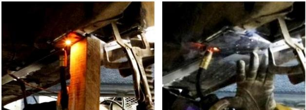
Figure 49 – Weld Doubler Plate
