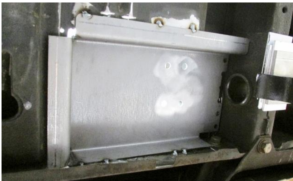
Figure 12 - Tack Weld Rear Mount
