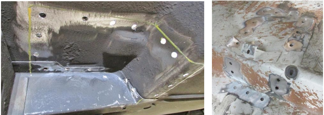
Figure 8 - Drill Plug Weld Holes
