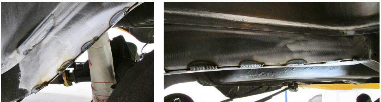
Figure 5 – Stitch Weld Inner Frame Rail Doubler (Driver Side)
