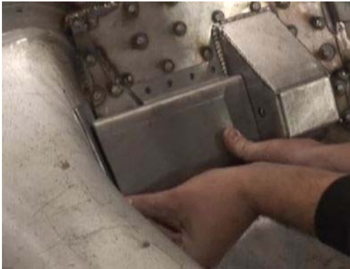
Figure 10 – Fit the Inner Brace and Tunnel Doubler
