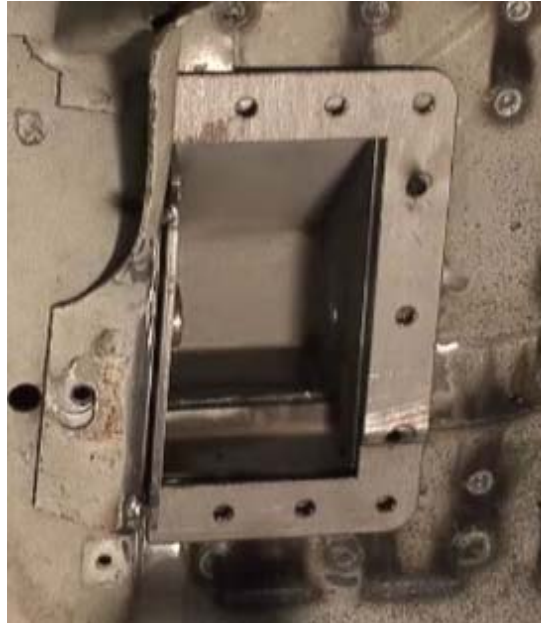
Figure 16 - Plug Weld Close-Out
