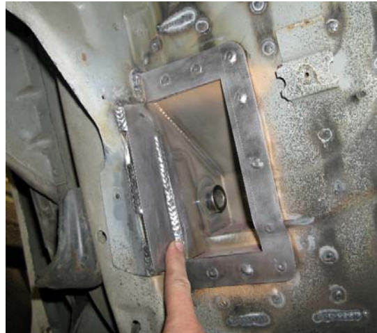
Figure 17 - Finish Weld Flange & Close-Out
