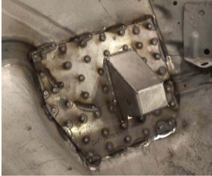
Figure 9 – Finish Weld Lower Doubler Plate
