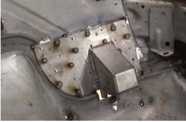
Figure 5 – Plug and Tack Weld in Place
