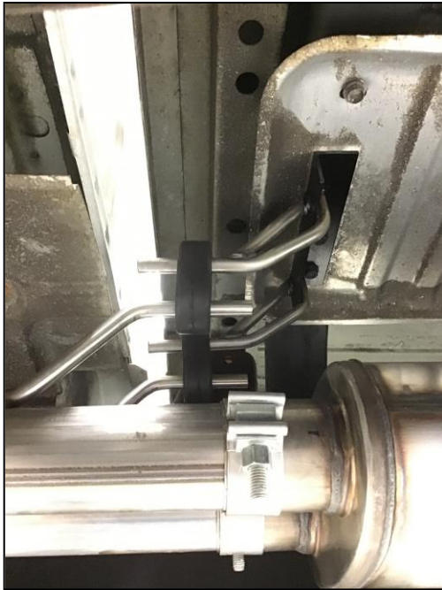
Figure 1 Before muffler hanger rod attachment to frame
