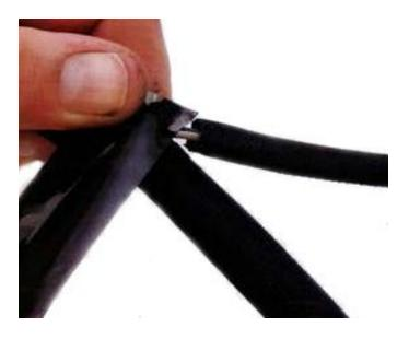
**Step Six:** Be sure to maintain tension on the tape while wrapping the breakout.
