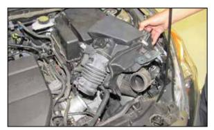
7. Lift up the air box to disconnect it from the mounting grommets, then disconnect the fresh air duct and remove the air box from the vehicle. **NOTE: K&N Engineering, Inc., recommends that customers do not discard factory air intake.**
