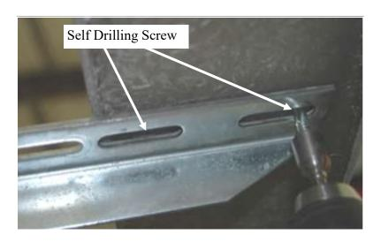
Using self drilling screws attach the board to the angle brackets making sure you are drilling into steel mounting pads. Level board and tighten any remaining loose bolts at this time.
