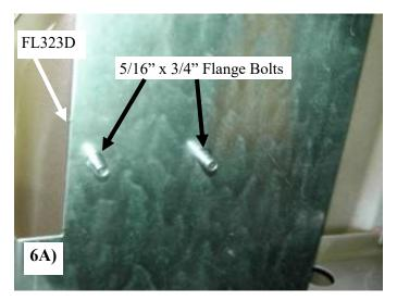
Place two 5/16" x 3/4" flange bolts down through the holes in the FL323D from the top, so the threads point downward shown in photo 6A
