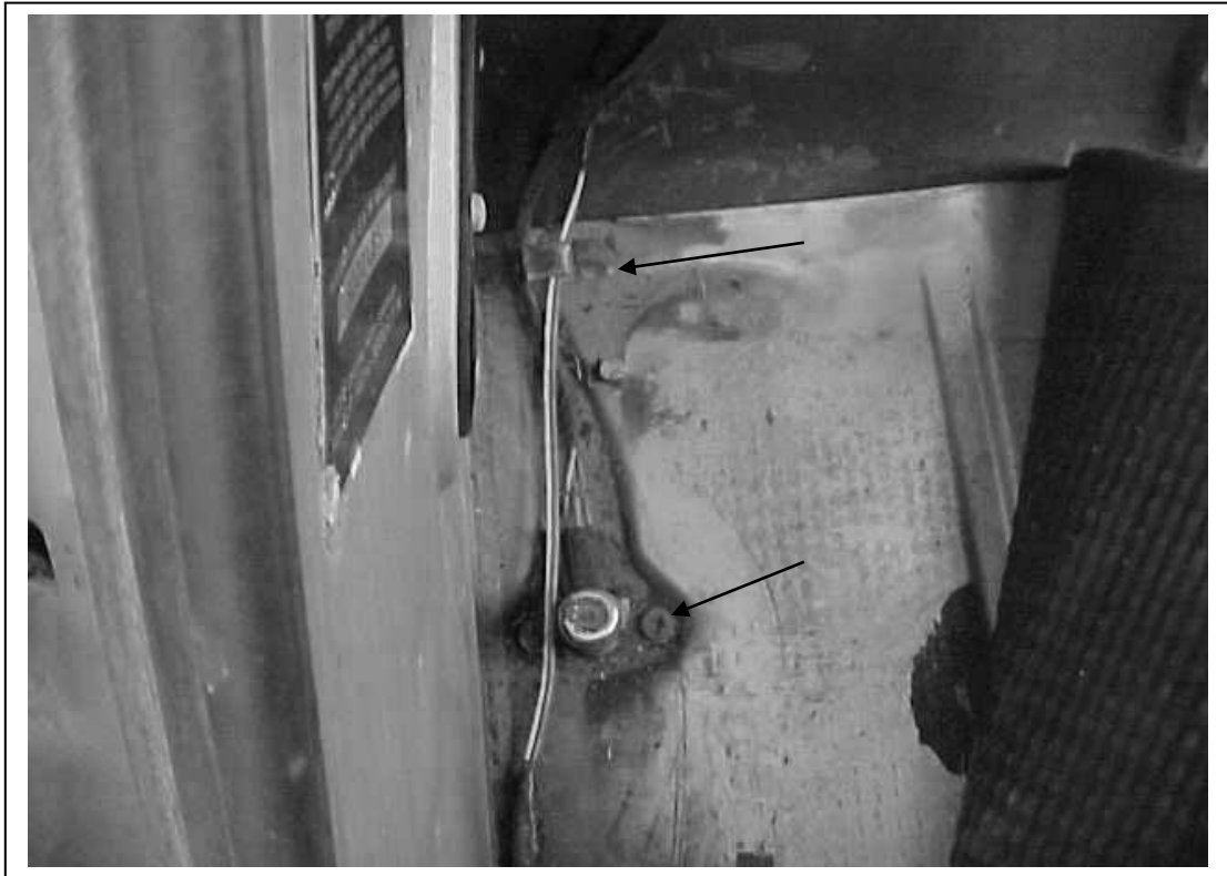
Figure 6.7 Routing of the Cab Section. Down from the fuse block and through the groove in the door jamb. Arrows are pointing at the Dimmer Switch and a mounting bracket.
