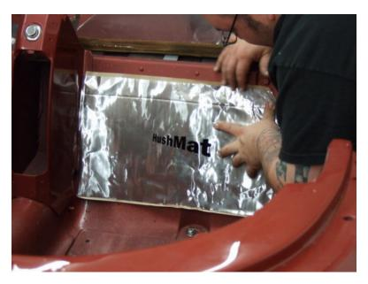
Take one sheet of the HushMat Ultra. Before removing the release paper place it onto the surface that you plan to install it. Make impressions in the foil of the sheet marking any cut outs that you will have to make.
