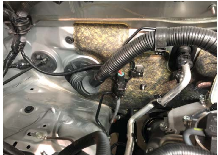
Wiring Harness Relocated
