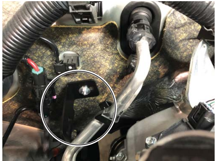
"L" Bracket Installed
