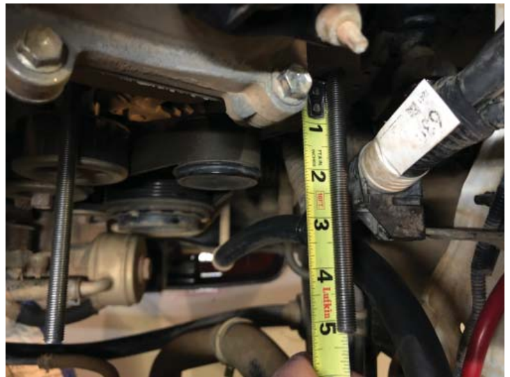
All Thread Installed
