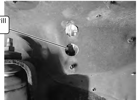
Wheel Well Side
