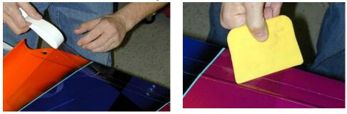
Surface Guard must be applied to a clean dirt free surface. A heavy duty scissors, knife or blade is necessary to cut Surface Guard. A squeegee should be used to spread out evenly.
