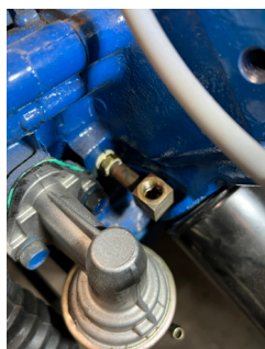
1/4" NPT extension pipe with 90 degree fitting installed.
