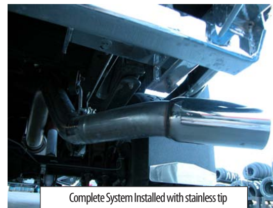
Complete System Installed
