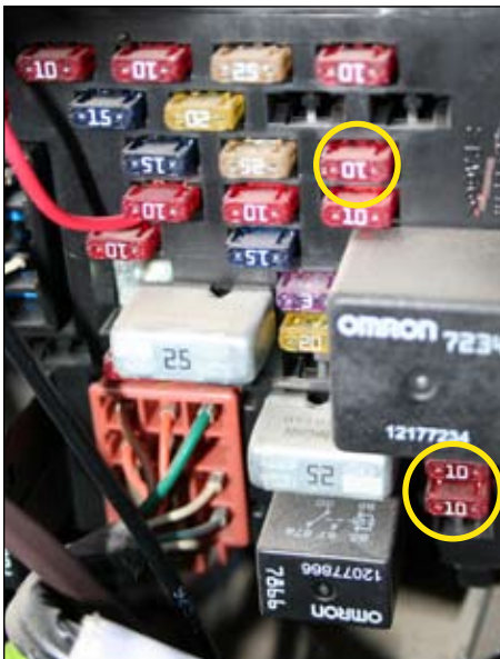
'01-'02 Interior Fuse Box
