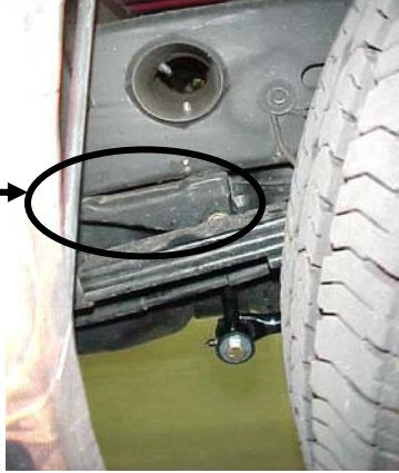
FRAME BRACKET MOUNTED ON THE DRIVERS SIDE.
