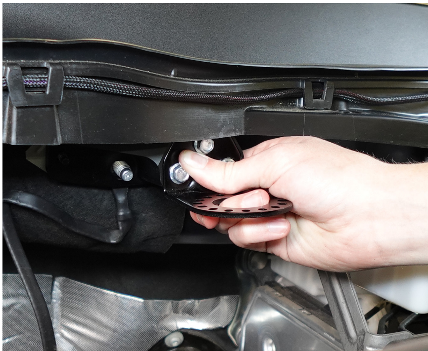
Figure 4 - Carrier Bracket Installed onto Firewall
