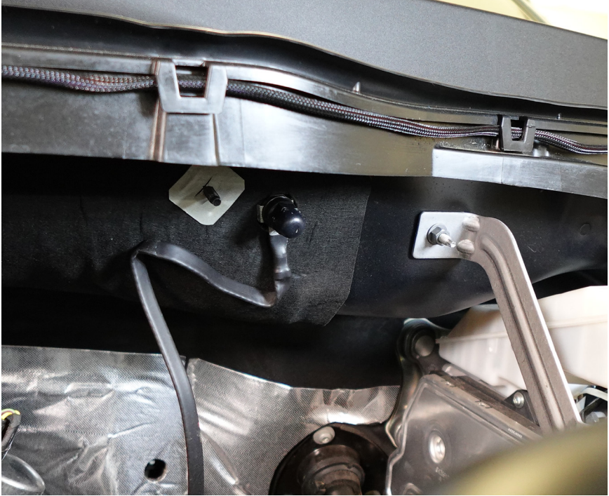
Figure 3 - Ground Wire Studs on Firewall
