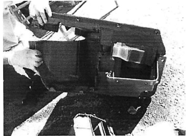
Step 9: With all hardware removed you can now separate the interior duct from the unit. Be sure to save all related pieces as they will be needed later in the installation.
