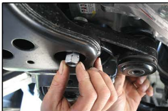
Fig. 8: Installation of Torque Arm Bracket
